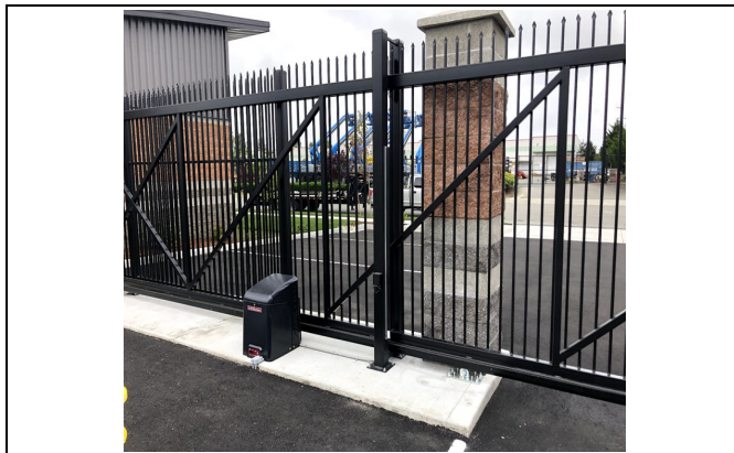
Public Safety Complex Gate
