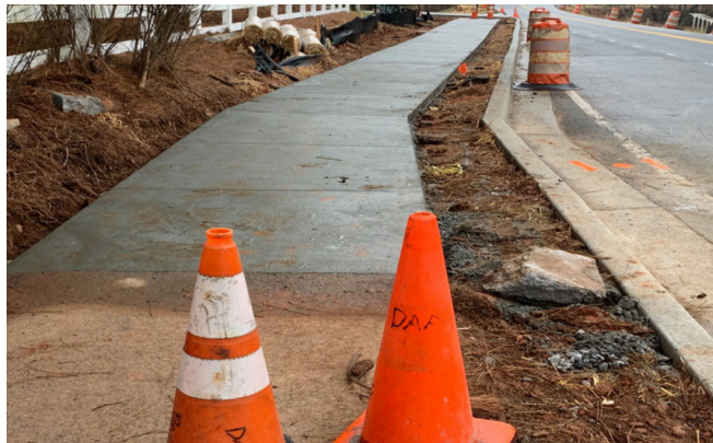
Sidewalk Repair and New Installation
