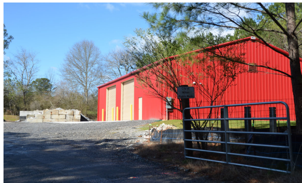
Public Works Yard
