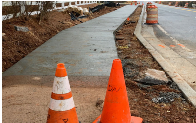
Sidewalk Repair and New Installation
