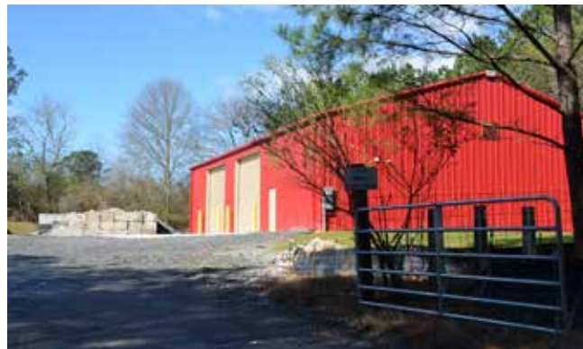
Public Works Yard
