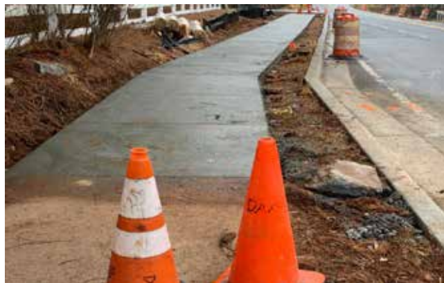
Sidewalk Repair and New Installation
