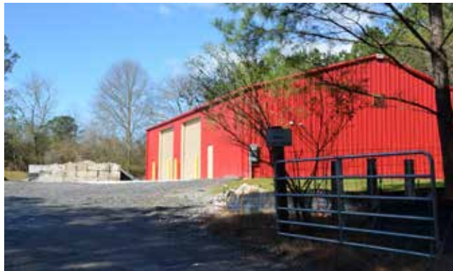
Public Works Yard
