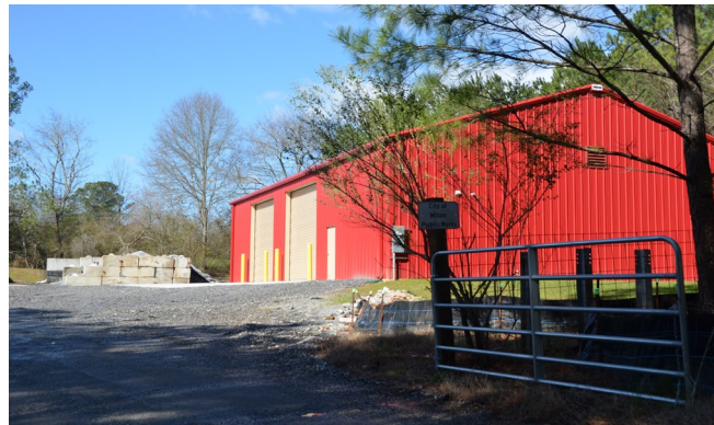
Public Works Yard
