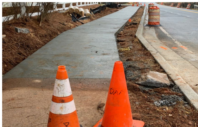
Sidewalk Repair and New Installation
