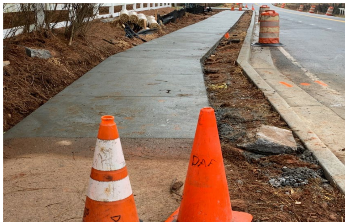
Sidewalk Repair and New Installation
