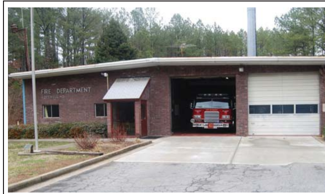
Fire Station 42 (15240 Thompson Road)
