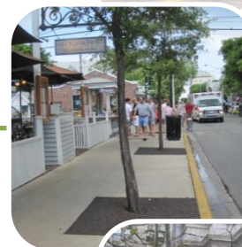
Key West, Florida uses permeable pavement as a surface over tree pits to protect tree roots from compaction while allowing for infiltration of water
