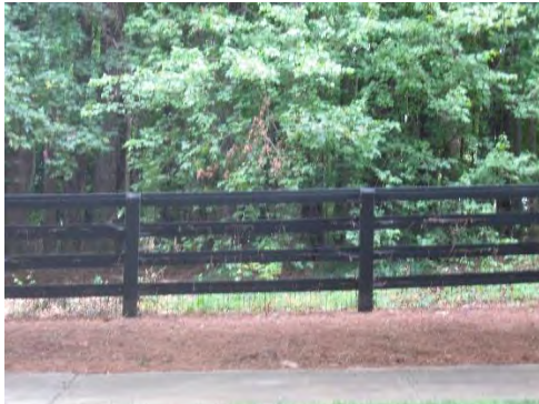
Photo 1. Four board fence along an exterior street.
