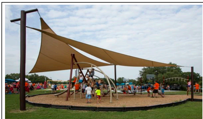
Example of shade structure
