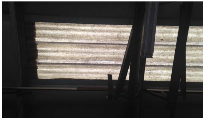
Station 42 Interior Sky Lights
