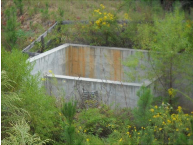
Overgrowth around outlet control box
