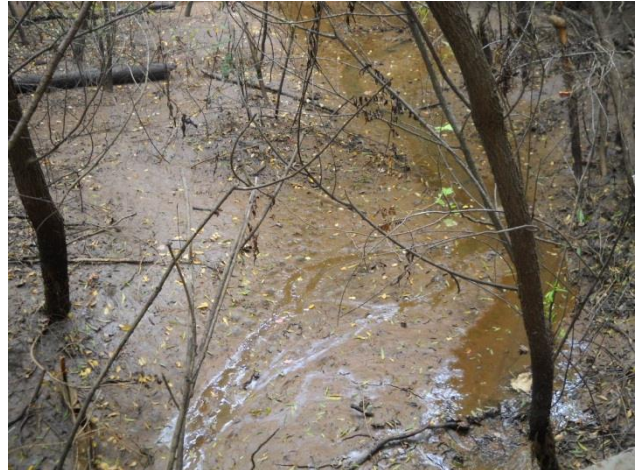
Accumulated silt and debris at bottom of pond
