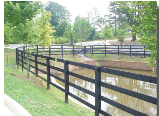
Black four-board fencing. See Section 31.
