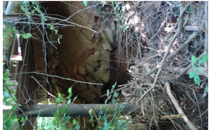
121-5010-0 – Substantial debris on creek channel
