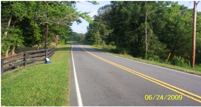
MLT06 – Roadway Northwest View
