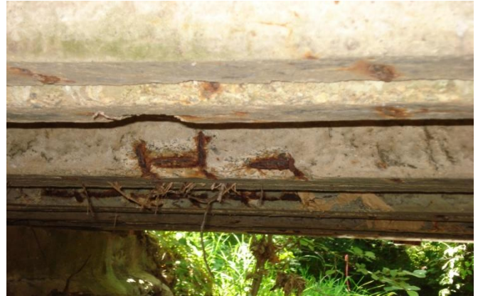
121-5008-0 – Underside Structure View
