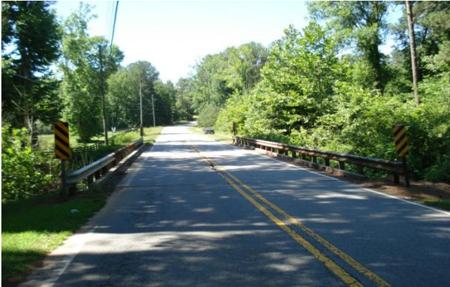
121-5009-0 – Roadway South View
