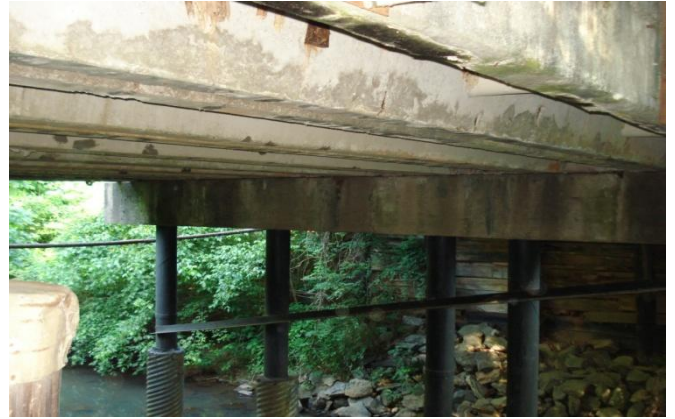
121-5011-0 – Underside Structure View
