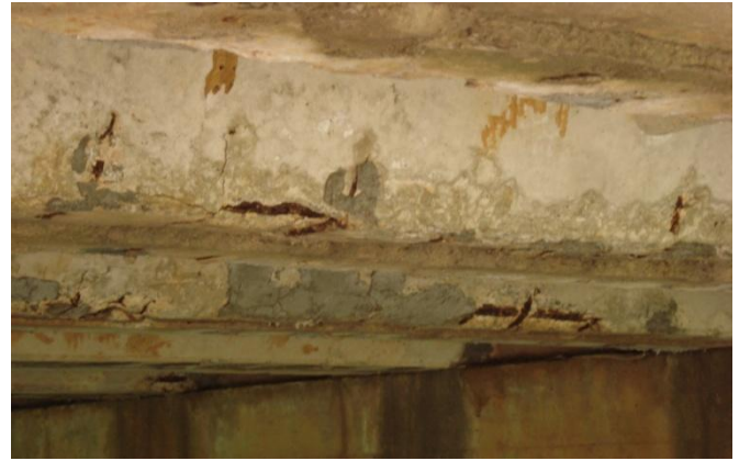
121-0284-0 – Significant spalling
