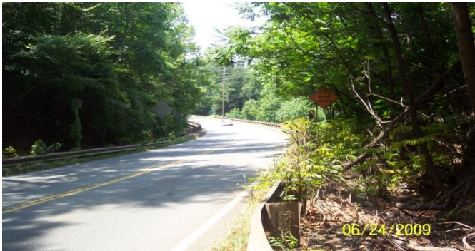
057-0029-0 – Roadway North View
