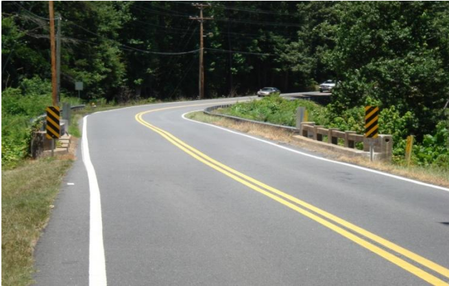
121-0283-0 – Roadway North View
