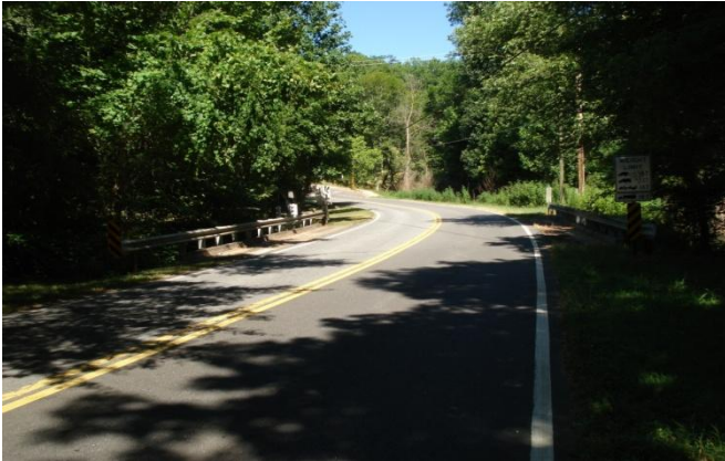
121-5010-0 – Roadway West View
