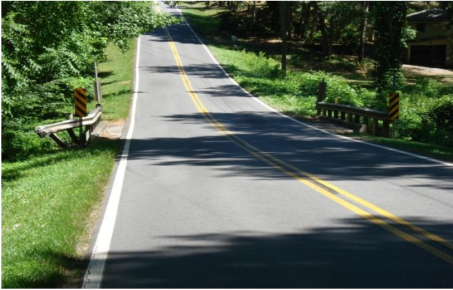
121-5202-0 – Roadway North View
