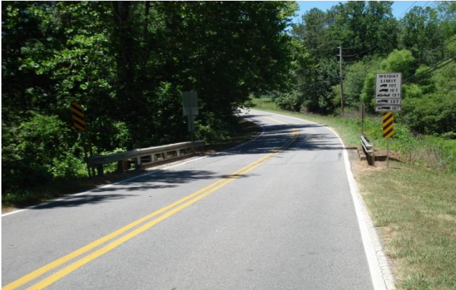
121-5003-0 – Roadway West View
