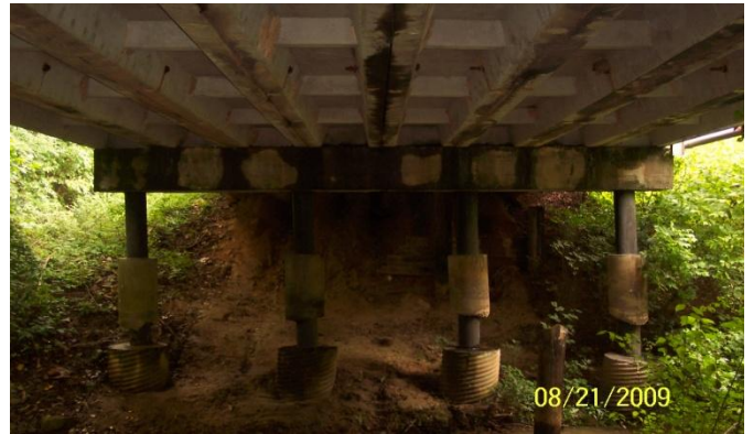
121-5151-0 – Pile Encasement at Bent 2
