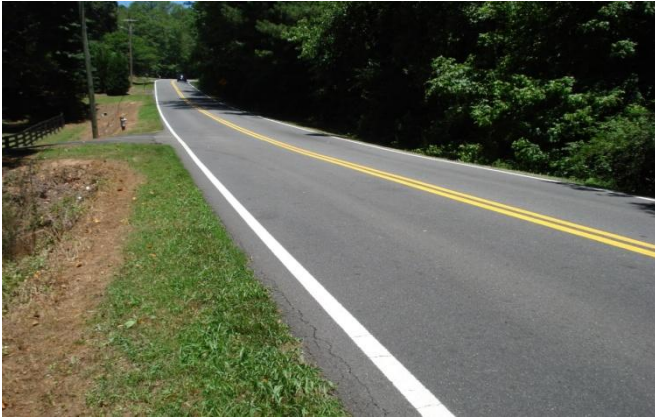
121-0282-0 – Roadway North View
