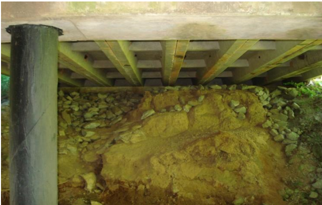
121-5004-0 – Underside Structure View
