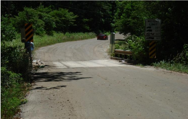
121-5008-0 – Roadway South View
