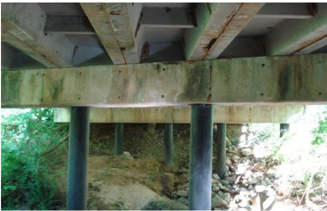
121-5013-0 – Underside Structure View
