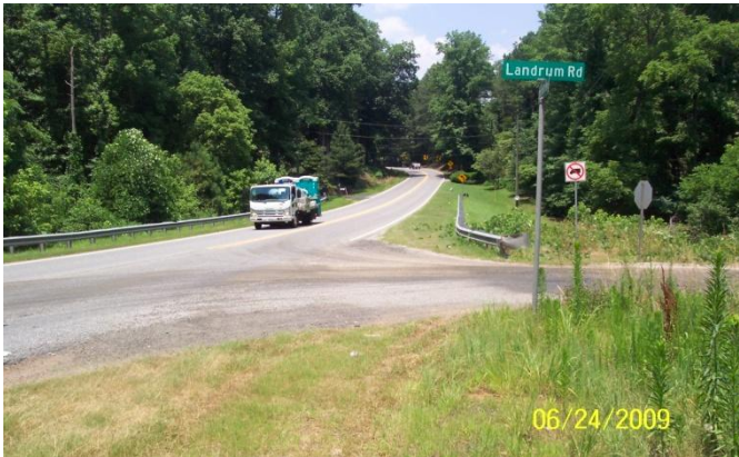
121-0697-0 – Roadway North View
