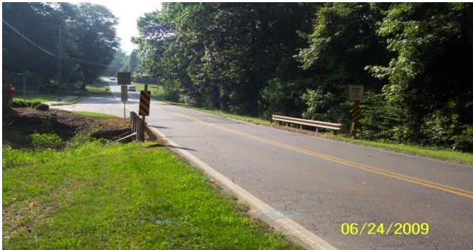
MLT04 – Roadway West View
