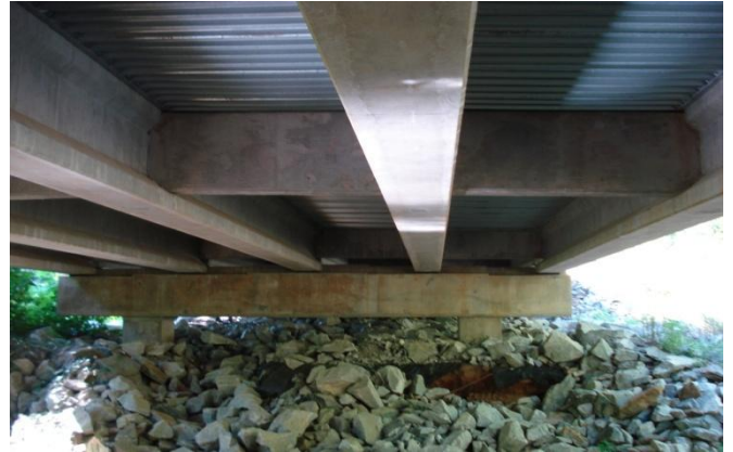
121-5303-0 – Underside structure View
