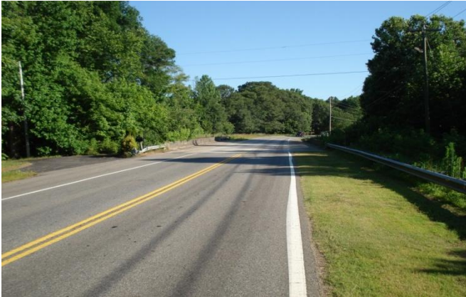
121-0698-0 – Roadway North View
