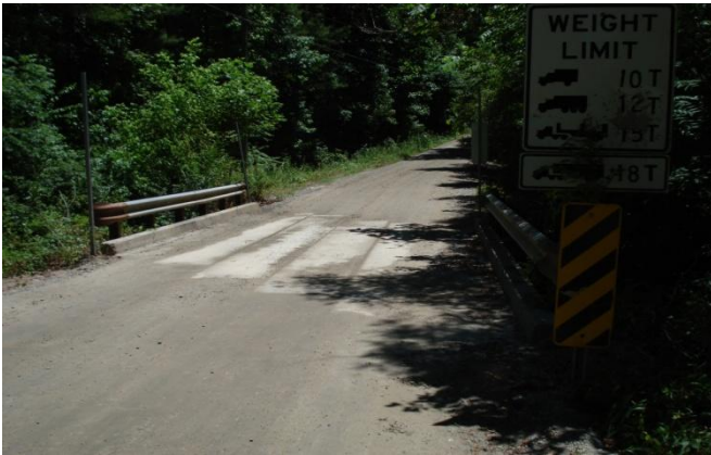
121-5007-0 – Roadway South View
