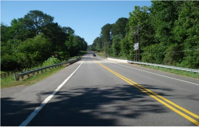
121-5303-0 – Roadway South View
