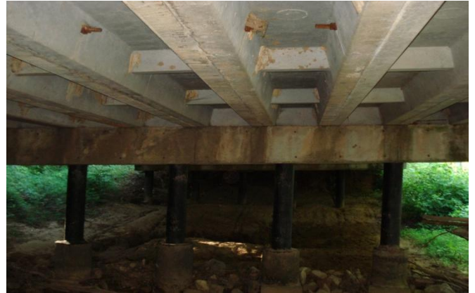
121-5012-0 – Underside Structure View
