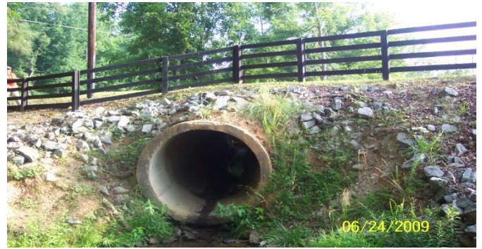
MLT06 – Outfall Elevation View
