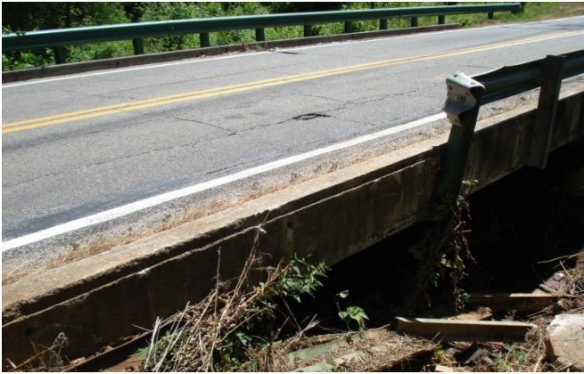
121-0284-0 – Damaged guardrail
