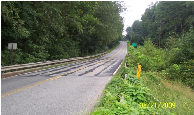
121-5151-0 – Roadway East View
