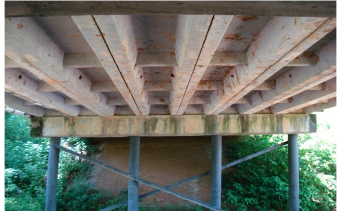
121-5006-0 – Underside Structure View
