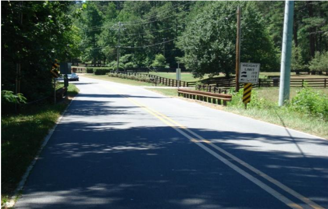
121-5004-0 – Roadway West View
