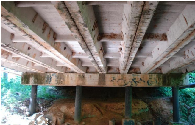
121-5009-0 – Underside Structure View
