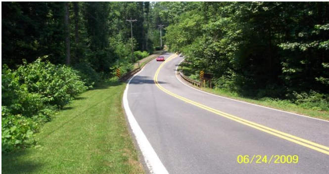
121-5015-0 – Roadway East View
