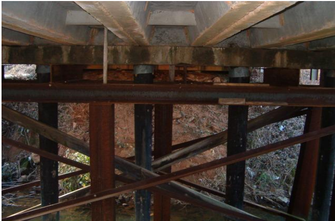
121-0281-0 – Substructure repairs in place
