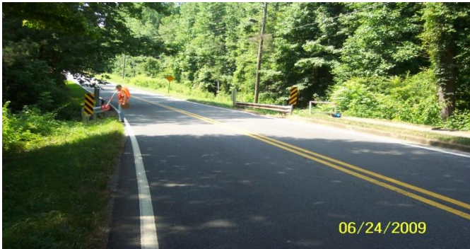
MLT01 – Roadway South View
