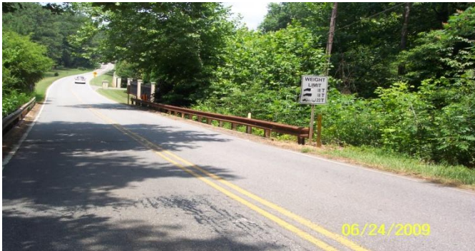
121-5153-0 – Roadway North View
