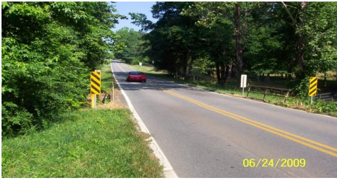
MLT05 – Roadway West View
