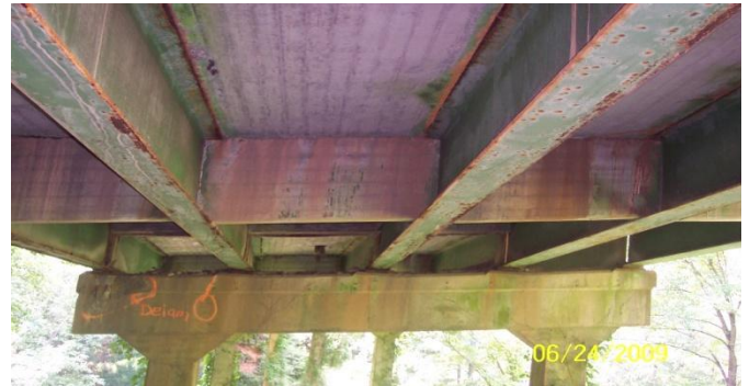
057-0029-0 – Bridge superstructure from below
