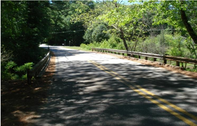
121-5006-0 – Roadway West View
