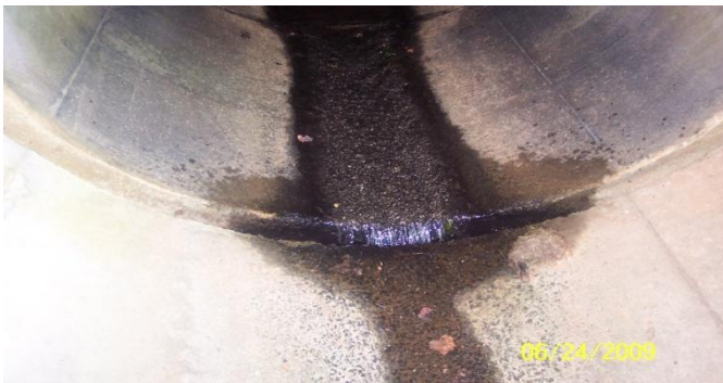
MLT06 – Last pipe segment at pipe outfall
