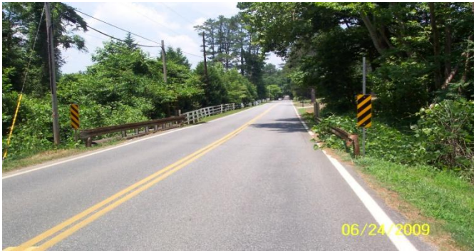
121-5016-0 – Roadway North View
