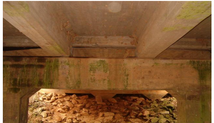
121-5106-0 – Underside Structure View
