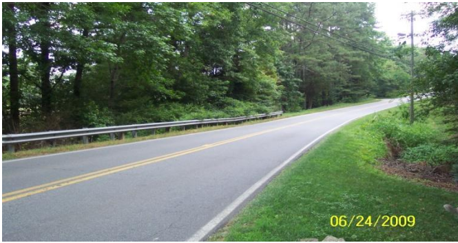
121-5107-0 – Roadway North View
