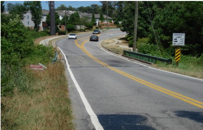
121-0284-0 – Roadway East View
