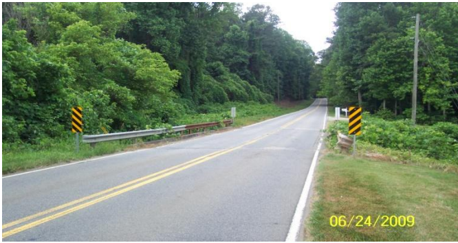
121-0281-0 – Roadway South View
