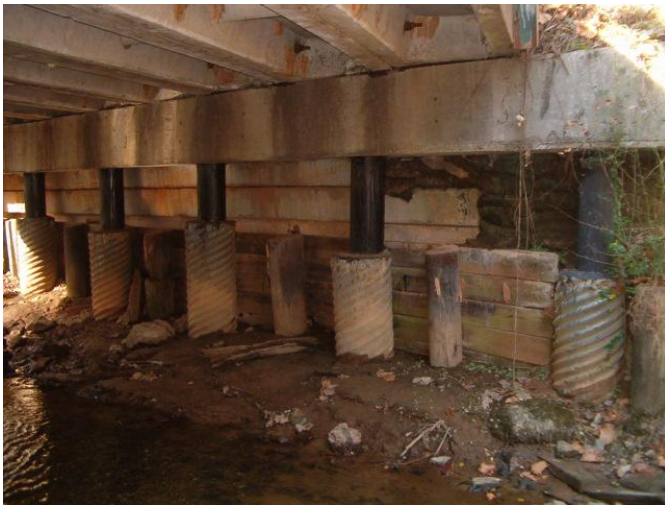
121-5016-0 – Substructure repairs in place
