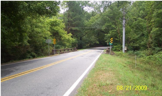
121-5106-0 – Roadway South View
