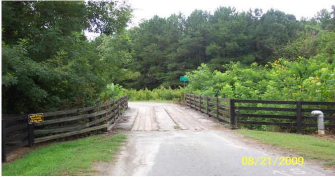
121-5002-0 – Roadway South View
