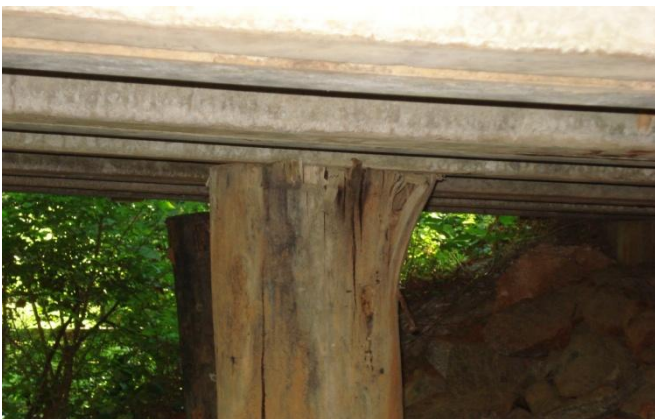
121-5014-0 Deck concrete panels bearing on pile
