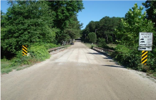
121-5013-0 – Roadway North View
