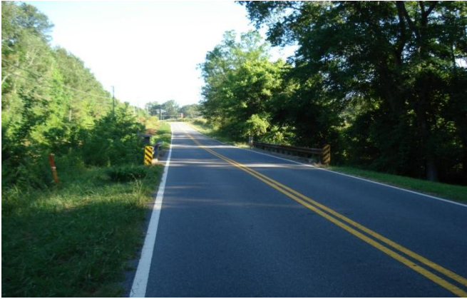
121-5011-0 – Roadway NW View
